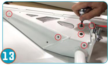
Attach latch plate to door using (4) provided bolts. Secure all 8 bolts from steps 4-6.
