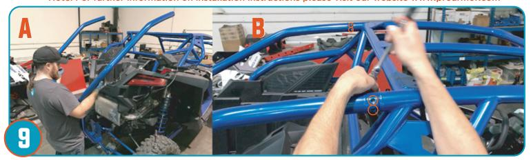
A. Place rear section of cage onto your Pro XP. B. Tighten 4 cage bolts joining the rear to the main section of the cage. Adjusting jack height up or down may assist in aligning the cage sections. Inside bolts thread from inside-out of cage tubing. Outside bolts thread from the outside-in.
