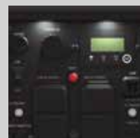
Illuminated Control Panel
